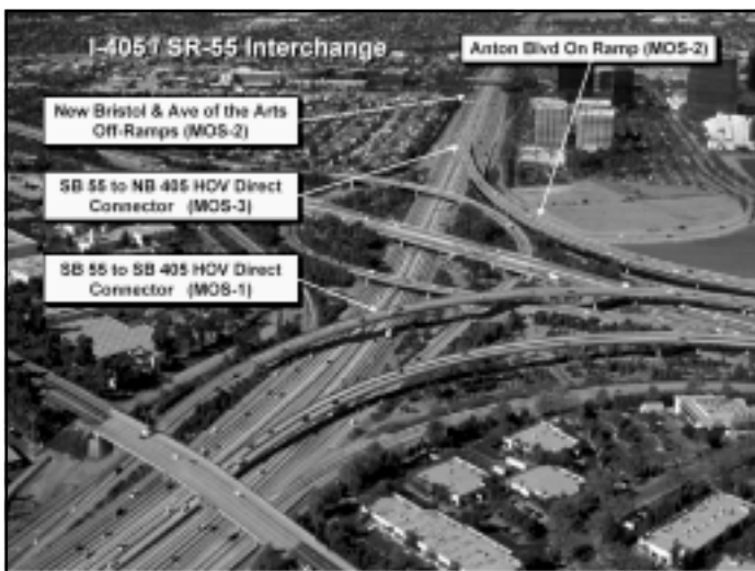
Figure 2: A New Freeway Interchange in Orange County Aims to Improve Traffic Flow in Airport/South Coast Plaza Area. Westbound view of the freeway intersection shown in Figure 1. MOS stands for minimum operating segment. As any other government agency, OCTA lives by its own acronyms.
